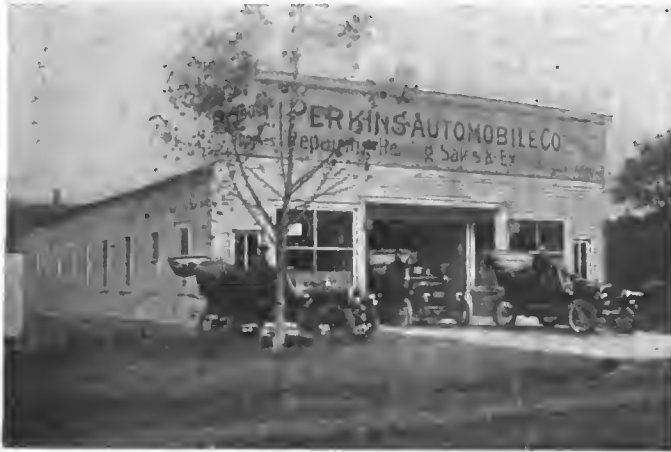
A MODERN GARAGE AT ROCKAWAY, NEW JERSEY.
